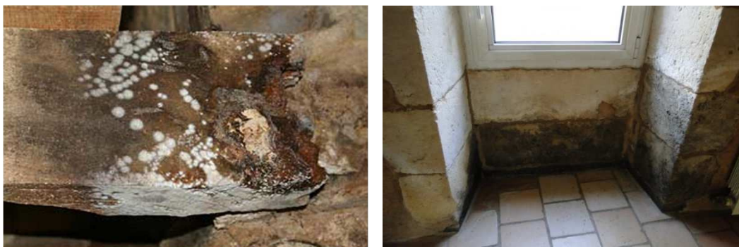
Figure 3 : Illustration of the technical stakes associated with the risks of pathology after energy retrofit (source: STBA)
