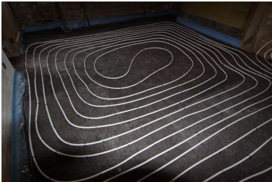
Figure 29 : Plancher chauffant
