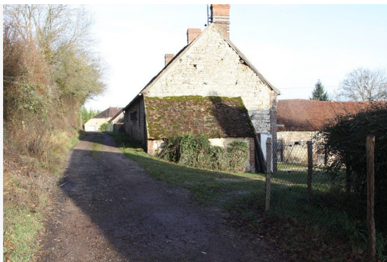
Figure 2 : Façade nord semi-enterrée
