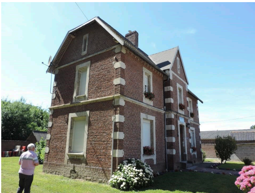
Figure 1: Exterior façades of the town hall of Brias
