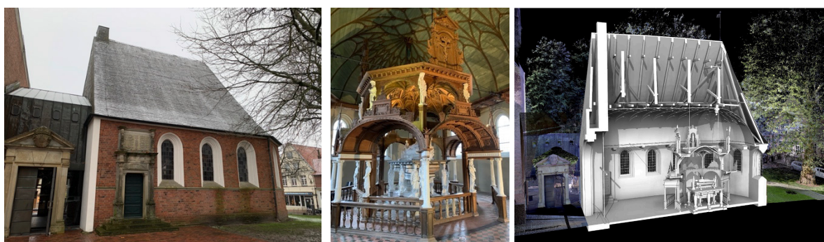
Figure 1. Exterior view (left), interior view (middle) and the point cloud based 3D-model (right) of the Edo-Wiemken-Monument in Jever (source 3D-model: DhochN-Nord Digital Engineering GmbH).
