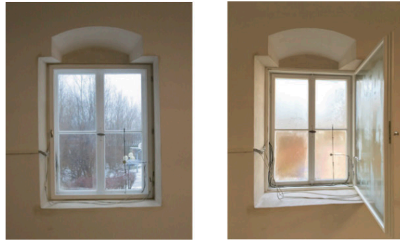
Figure 4. Interior view of window 1.27 with closed (left) and open inner window casement. A heat flow sensor can be seen in the middle of the lower right glazing.
