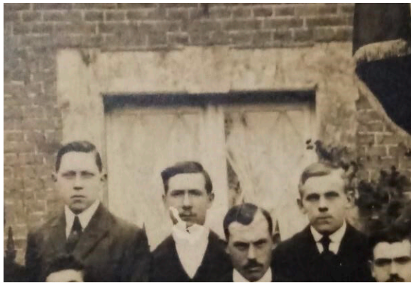
Figure 2: Original appearance of the windows
