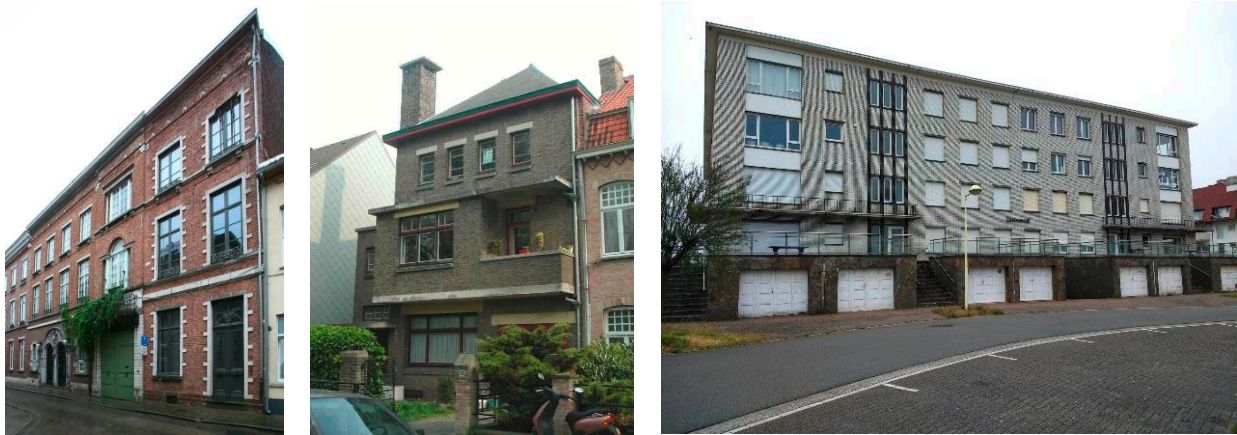
Figure 1. Three case-studies: 19 th century mansion (Diest), House ‘Billiet’ (Bruges), Residence ‘Duinpark’ (Koksijde)
