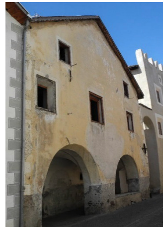
Figure 2 Reference building of Climate zone II (Portici house-II), Schallerhaus, Glorenza
