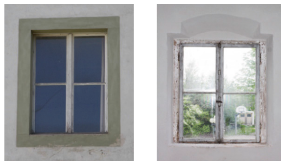
Figure 3. Old Cooperage upper floor, window 1.26 on the north side with exterior and interior views, historic casement window in its original state. Frame dimensions 1.14 m x 1.40 m (1.60 m 2 ).
